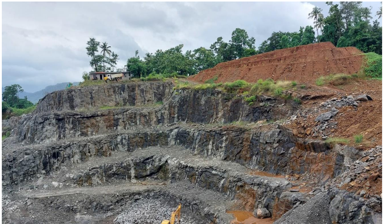
PHOTOGRAPHS SHOWING FORMATION OF BENCHES
