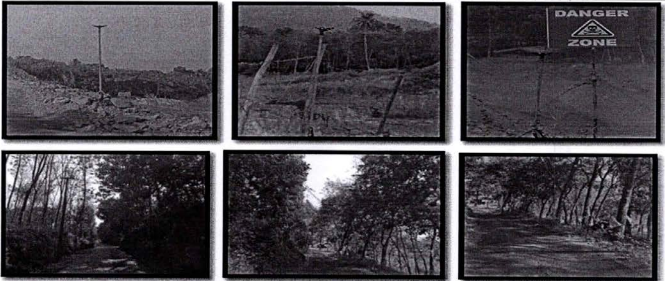
Fig 11-13: Sprinklers for Dust Suppression and Fig 14-16: Approach and Internal Roads
