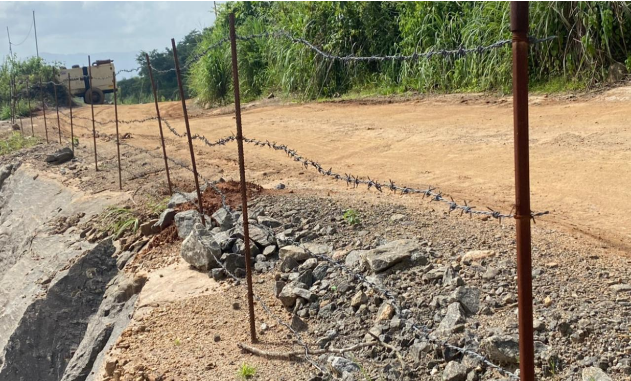
PHOTOGRAPHS SHOWING THE FENCING AROUND THE QUARRY
