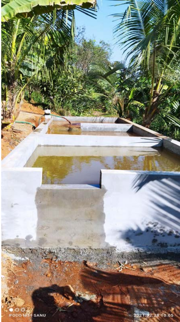
PHOTOGRAPHS SHOWING NEWLY BUILD RAIN WATER HARVESTING STRUCTURE
