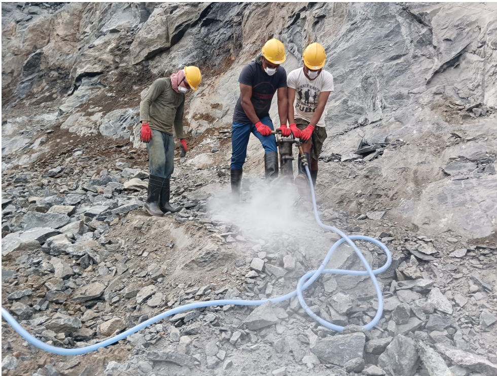
Photograph showing the workers wearing PPE's
