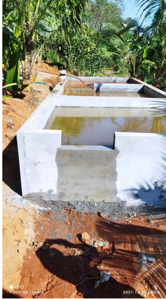
PHOTOGRAPHS SHOWING NEWLY BUILD RAIN WATER HARVESTING STRUCTURE
