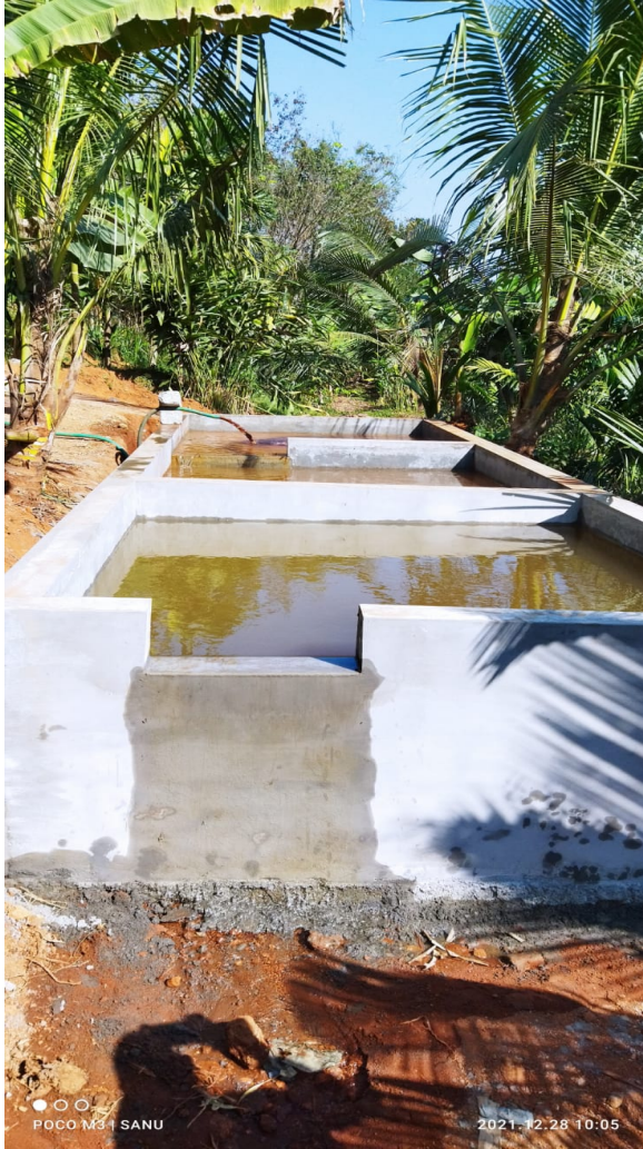
PHOTOGRAPHS SHOWING NEWLY BUILD WATER SETTLING TANK FOR GROUND WATER RECHARGE
