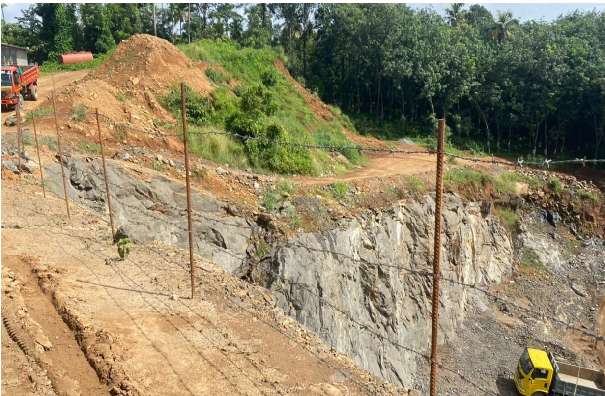
PHOTOGRAPHS SHOWING THE FENCING AROUND THE QUARRY
