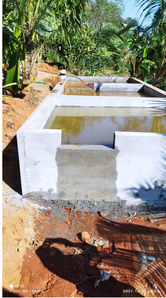
PHOTOGRAPHS SHOWING NEWLY BUILD WATER SETTLING TANK FOR GROUND WATER RECHARGE
