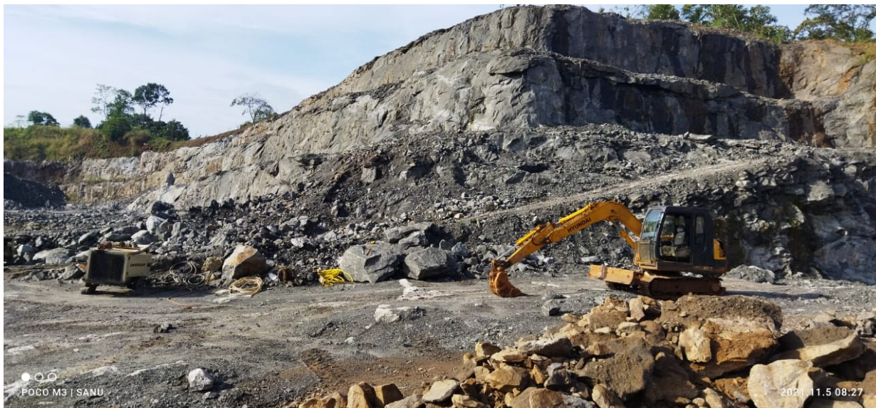
PHOTOGRAPHS SHOWING FORMATION OF BENCHES
