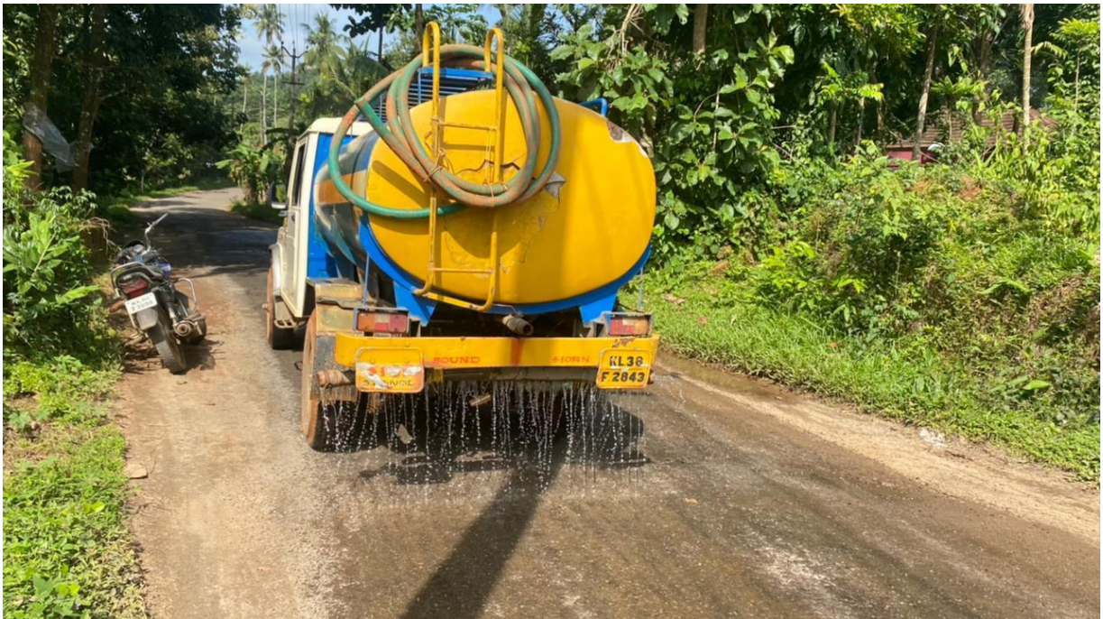
PHOTOGRAPHS SHOWING THE WATER TANKER USED FOR SPRINKLING WATER FOR DUST SUPPRESSION
