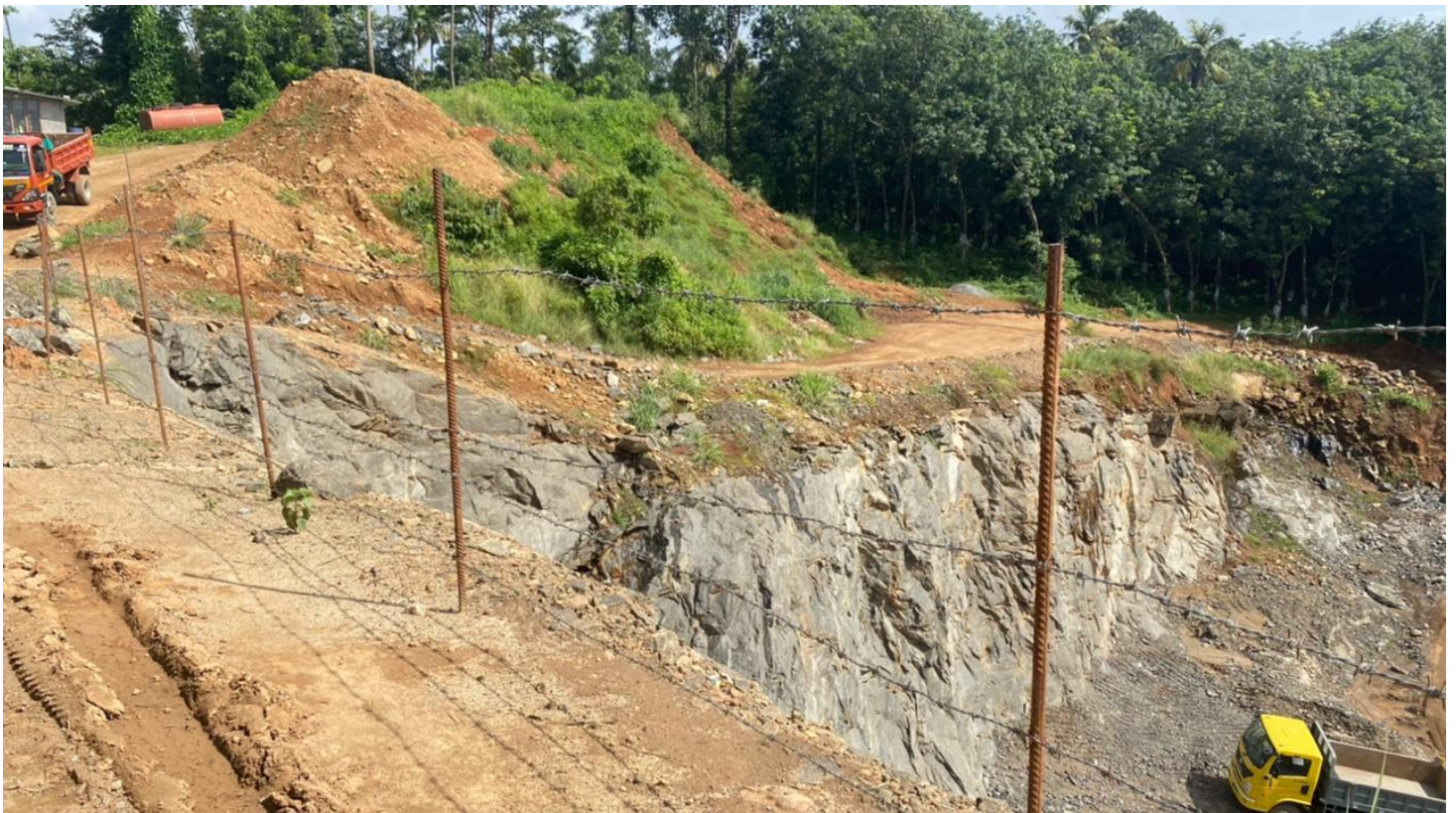
PHOTOGRAPHS SHOWING THE FENCING AROUND THE QUARRY
