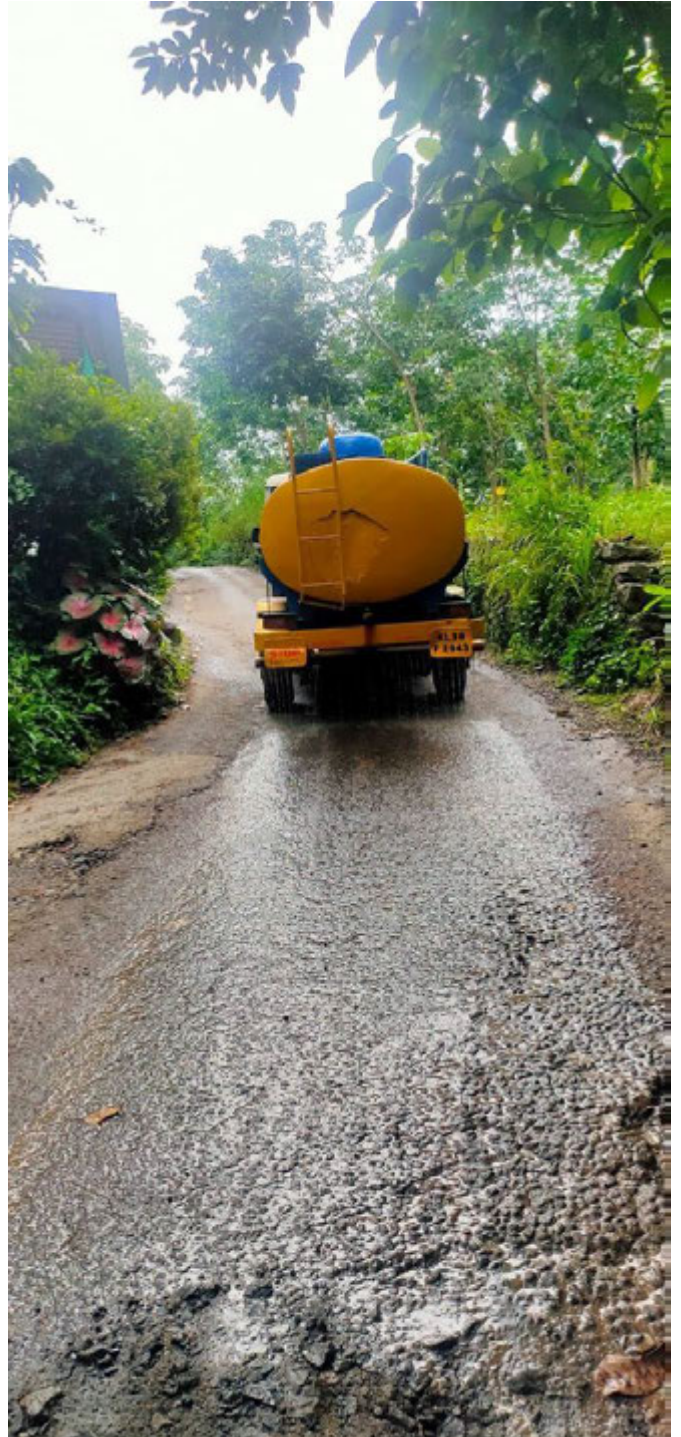
PHOTOGRAPHS SHOWING WATER SPRINKLING USING TANKERS FOR DUST SUPPRESSION
