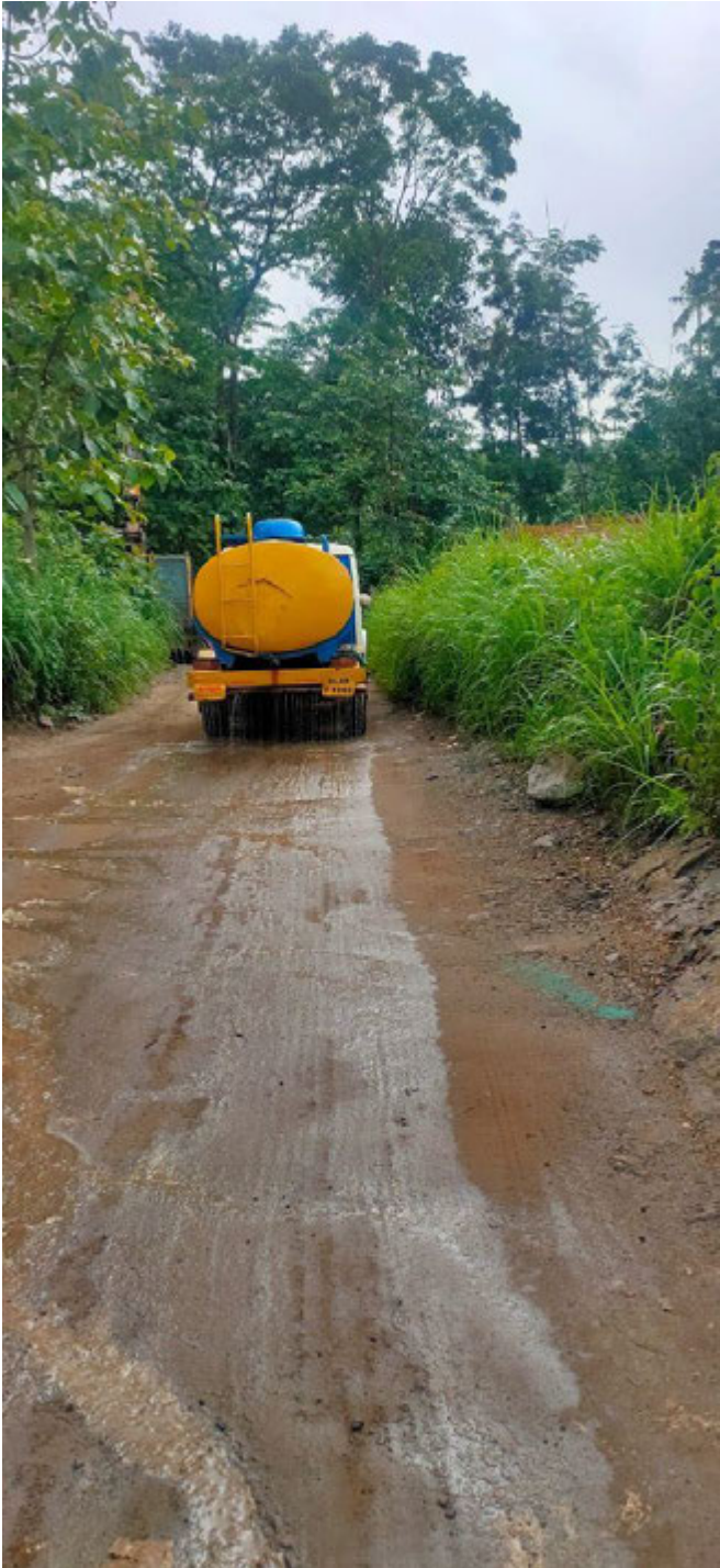
PHOTOGRAPHS SHOWING WATER SPRINKLING USING TANKERS FOR DUST SUPPRESSION
