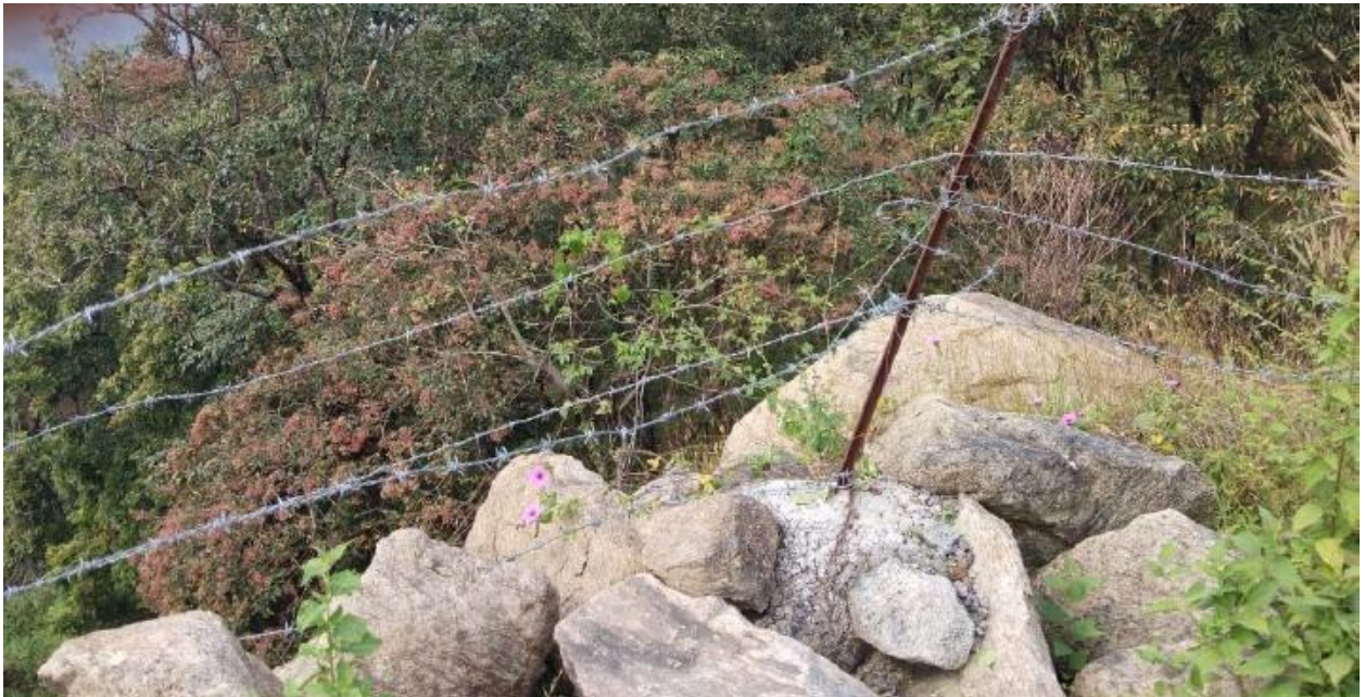
PHOTOGRAPHS SHOWING FENCING WITH BARBED WIRES
