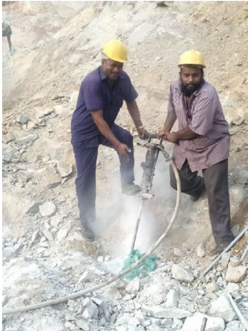
Photograph showing the workers wearing PPE's
