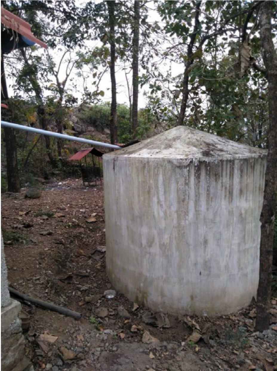
Photograph showing the rainwater harvesting tank
