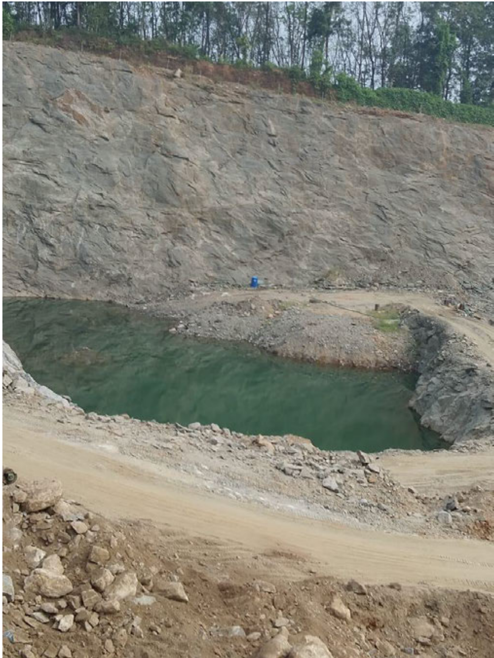
Photograph showing the excavated pit retained as rainwater storage pond
